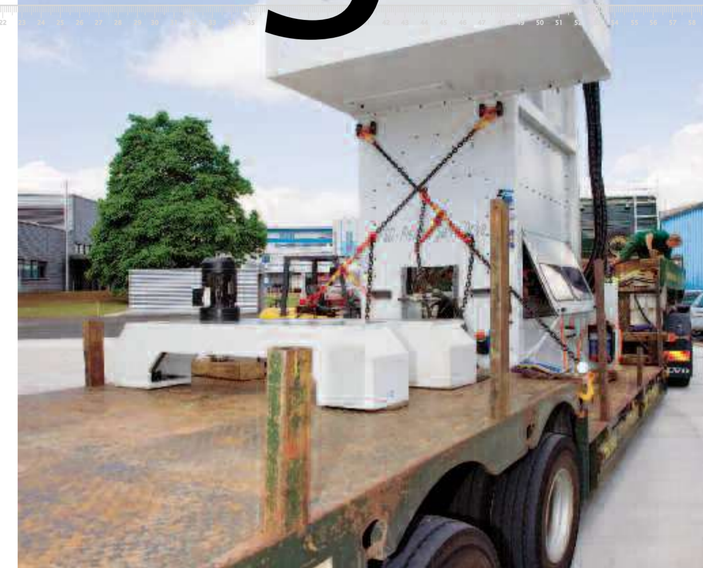
Relocating 60 tons – grand logistic performance.
